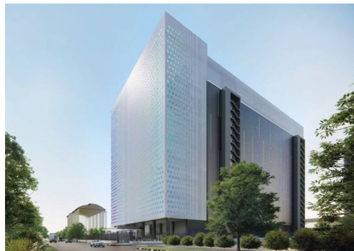
DC Tuas, Singtel Group's next-generation AI-ready and energy-efficient data centre
