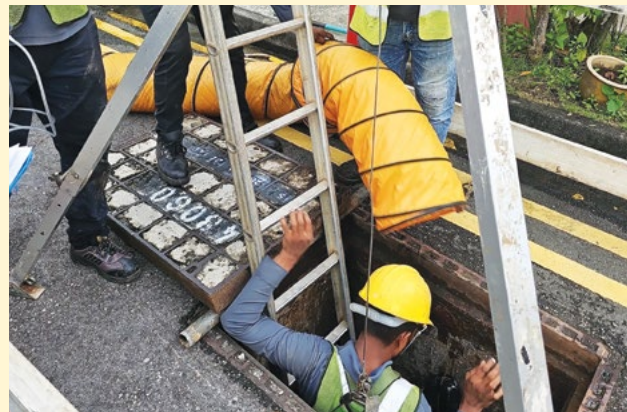
Prioritising safety in every manhole entry through checks, precautions and teamwork
